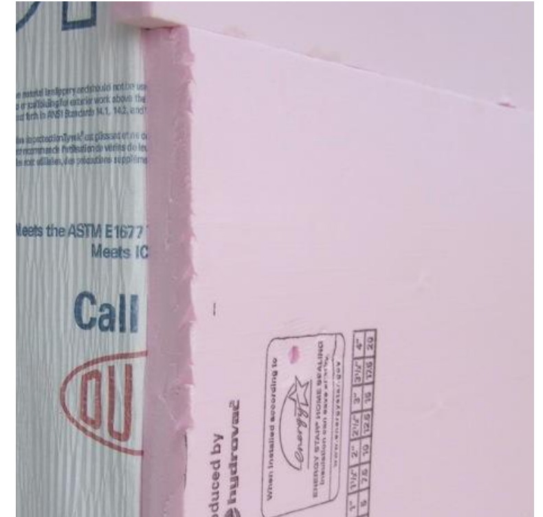
Add continuous insulation
