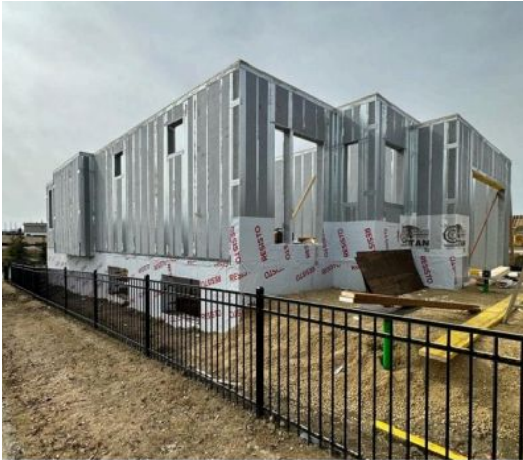
Figure 3 - ICE panels during erection
