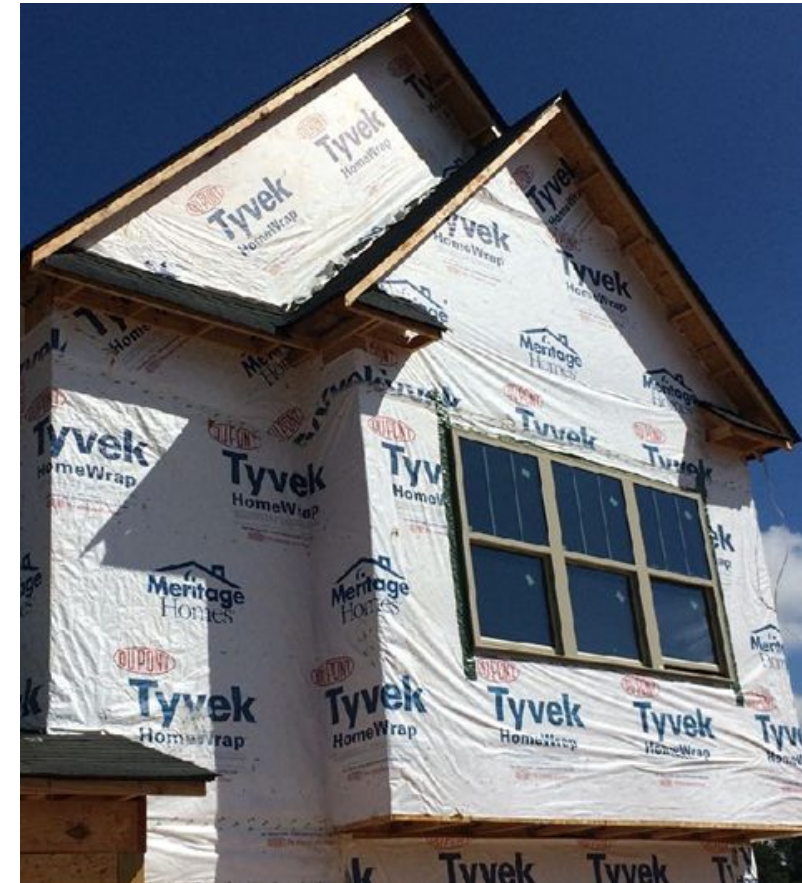
House Wrap Approach
