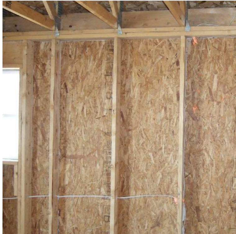
Reduce thermal bridges - Reduce framing
