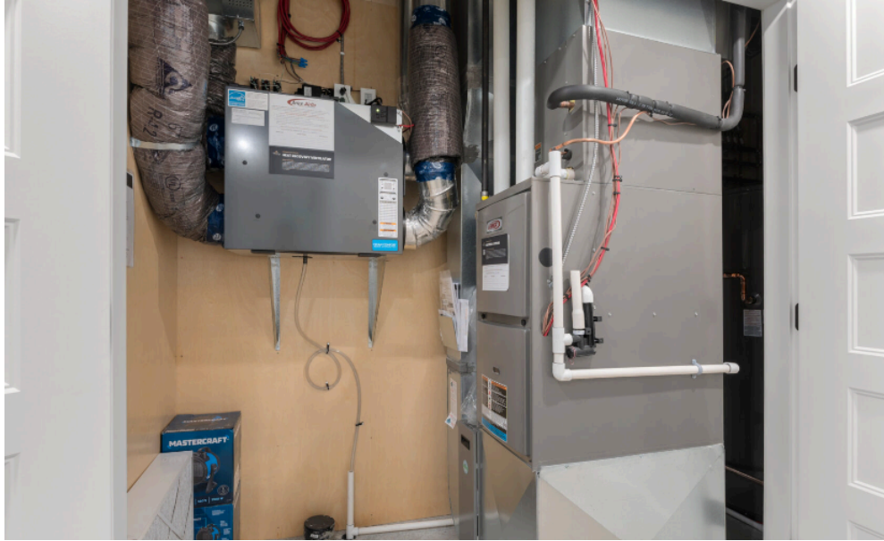
Figure 8 - Lennox ML296XV AUFE 96% natural gas condensing furnace, ECM motor with steam humidifier
