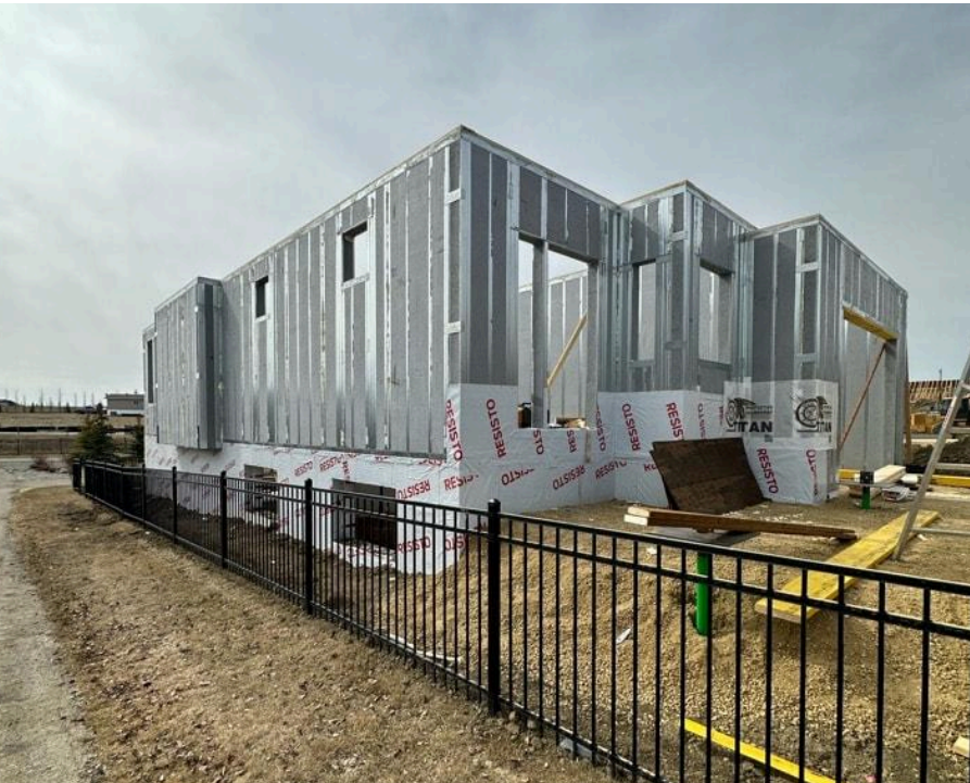
Figure 3 - ICE panels during erection
