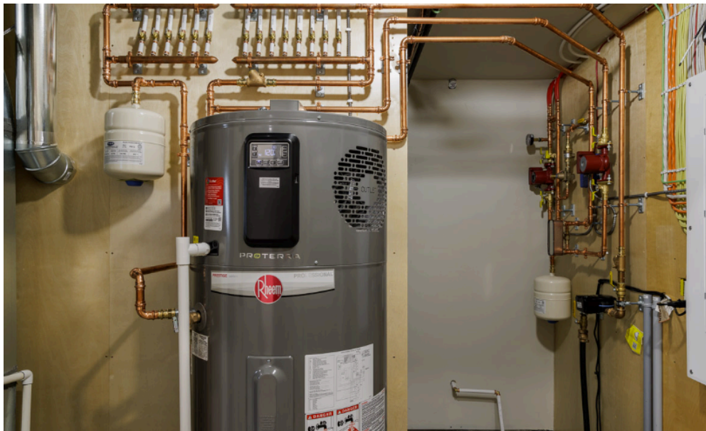
Figure 9 - Rheem Proterra Integrated heat pump (hybrid) hot water tank
