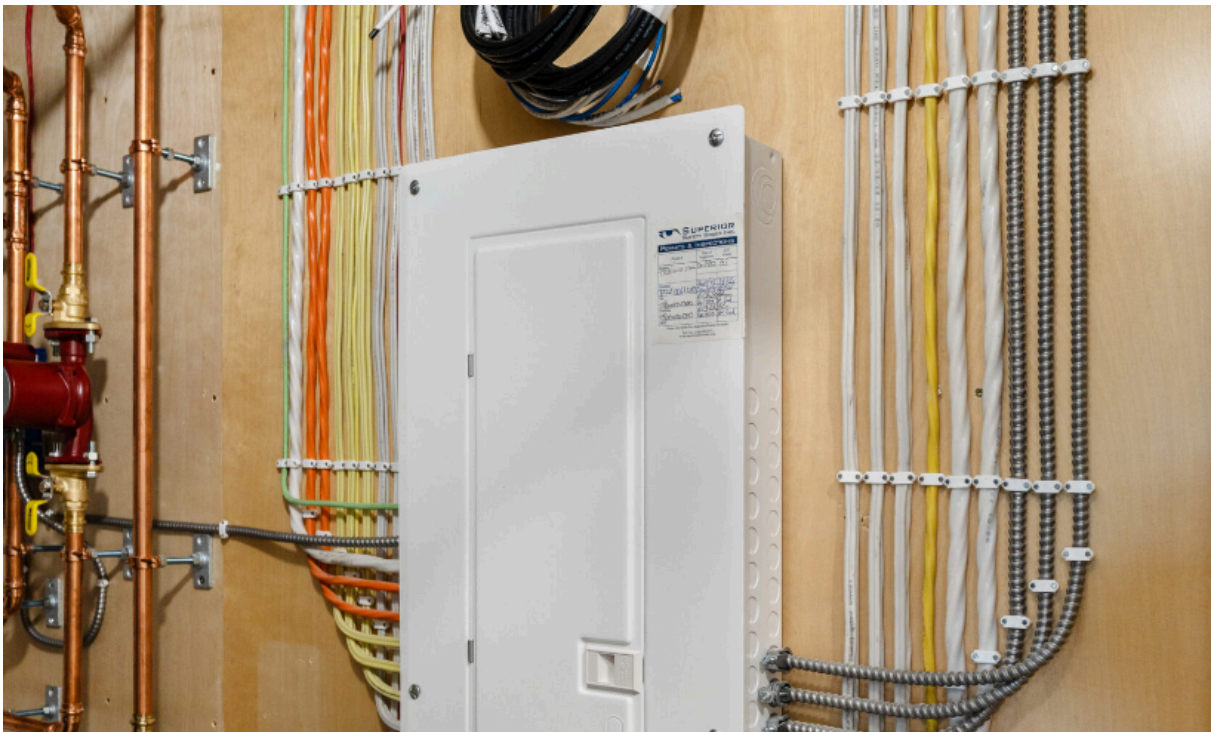
Figure 11 - Electrical panel with neatly organized wiring and conduit
