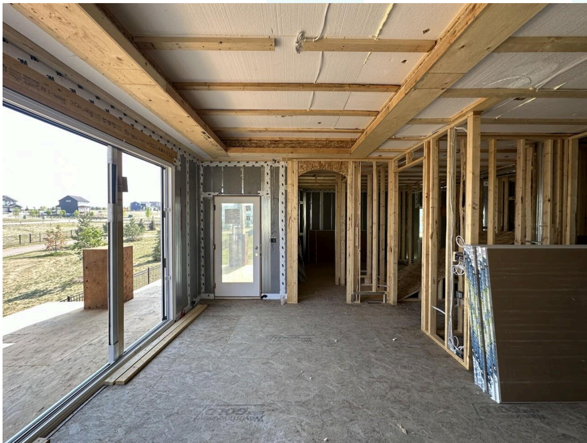
Figure 5 - 4” rigid EPS hung below the roof truss system
