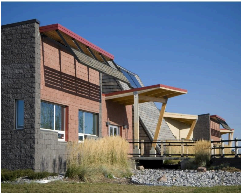
South exterior view of the Yellowhead County Administration Building, showcasing its mass timber design elements and architecture.
